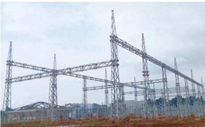
Design supply and fabrication and construction installation 150kV (7 bays) New Cianjur Substantion c/w 2 incomer dead end T/L tower and Mechanical electrical instalation.
