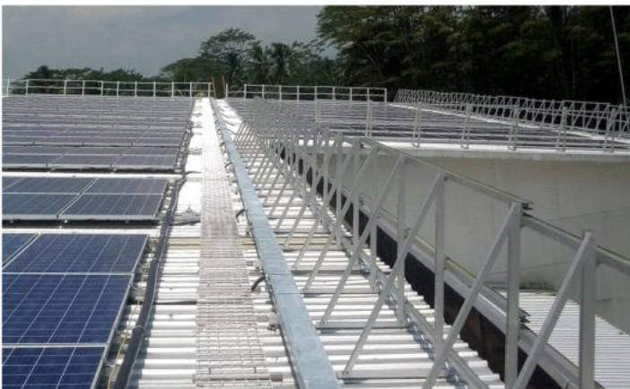
Ladder Platform for Solar PV Module instalation on rooftop - PT. Greenfield, Malang.
