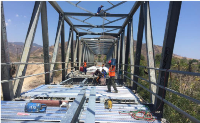
Jembatan flores 1 x40m & 1x55m reinforcement trust bridge ( design & fabrication & Construction supervision) Satker PU NTT.
